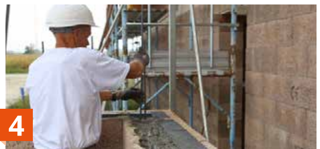
4 Fresh casting insertion of vertical seismic steel reinforcements
