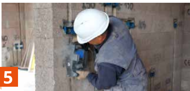
5 Chasing of wall with a router
