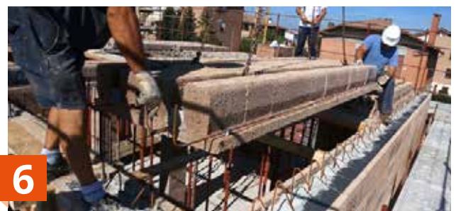
6 Laying of the floor slabs, calculated and made to measure.
