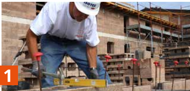
1 Laying of the first row with spirit level for levelling
