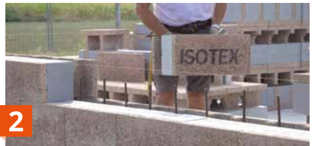
2 All subsequent rows laid dry
