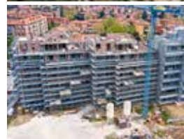
Multi-floor buildings in Bologna
